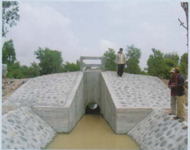
Secondary canal intake pipe culvert structure after construction
