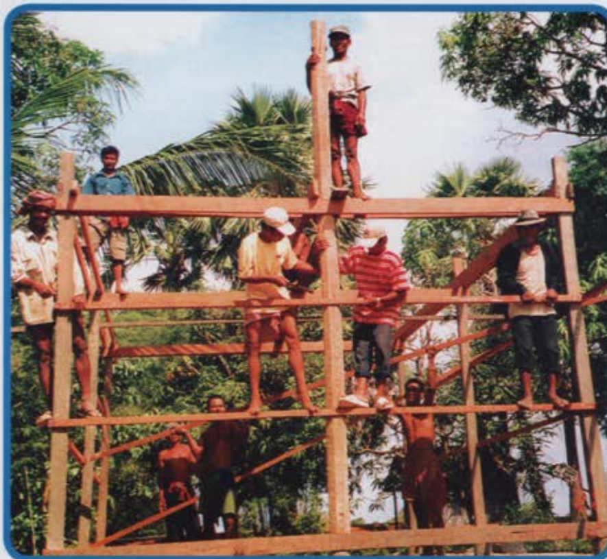
▲ Villagers working together to build the Community Fisheries Office
