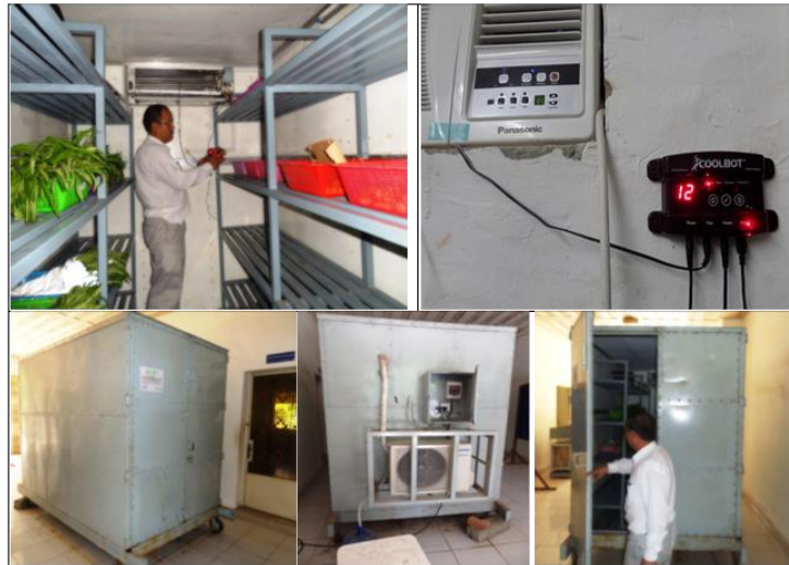
រូបភាពទី២០ Coolbot cold storage with the Coolbot device connected to the air conditioner.
