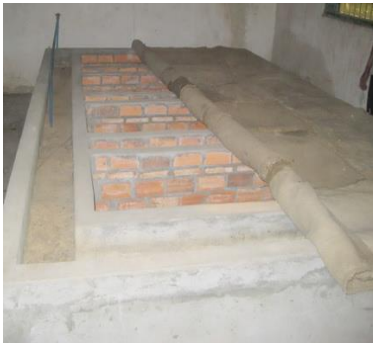
Brick-walled EC 4.5x2.5x0.6 m in length, width & height, 15–20 cm double wall with moist sand insulation
